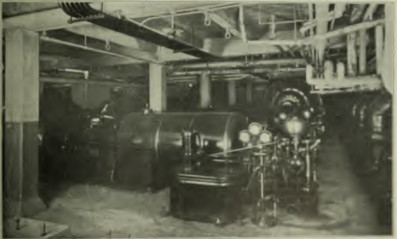
FIG. 1 THE TURBINE WITH MILWAUKEE PUBLIC SERVICE BUILDING.
